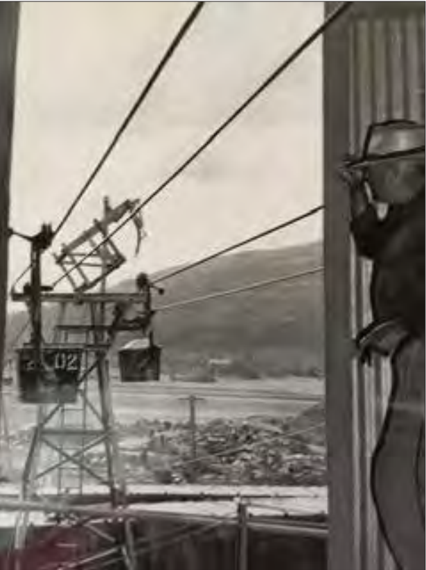
This photo shows a section of the tram carrying ore from the quarry to the magnesite plant south of Chewelah. Courtesy photo
