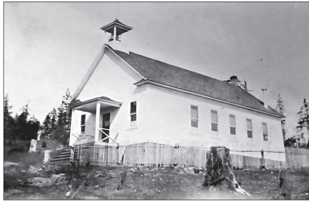
CAMANO CITY SCHOOLHOUSE FOUNDATION
