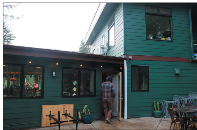
Chuck Stoltz, co-owner of Acorn & the Oak, walks into the restaurant-flower shop on Friday, Jan. 21, 2022. Stoltz and his wife, Janessa Stoltz (not pictured) hope to build a partially covered outdoor dining area on the roof of their Camas business.
