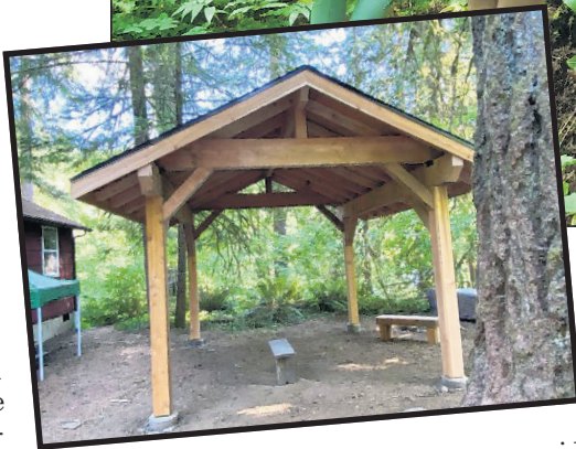
A Vancouver construction firm built a new wooden shelter at TreeSong Nature Awareness and Retreat Center in August 2021.
