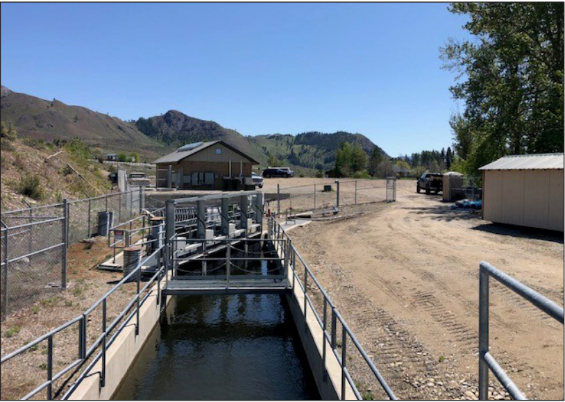
Photo Courtesy of Trout Unlimited A pumping station was installed at the new Barkley ditch headgate as part of a project to enclose open ditches on the east side of the Methow River.
