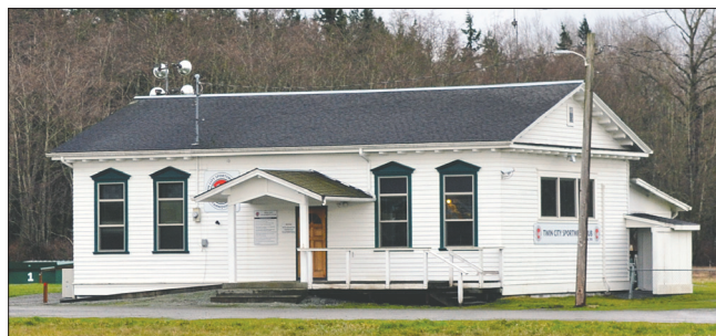
The original Irvine Library building was sold to the Twin City Sportsmens Club in 1970 and moved east of downtown on 64th Ave. NW, where it still stands.
