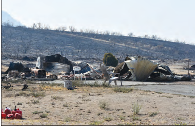
BROCK HIRES | The Chronicle Twisted metal and rubble are all that remain of a home in the Malott HUD housing development.
