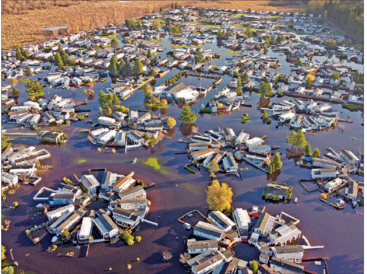
▲ November 15 flooding forced evacuations at Birch Bay Leisure Park on Birch Bay Drive. At least 20 residents in the 718-unit seasonal park were evacuated by park maintenance crews and as of November 21 were unable to return to their homes while the park continued to assess electric and sewer impacts. Photographed is residual water on November 19.
