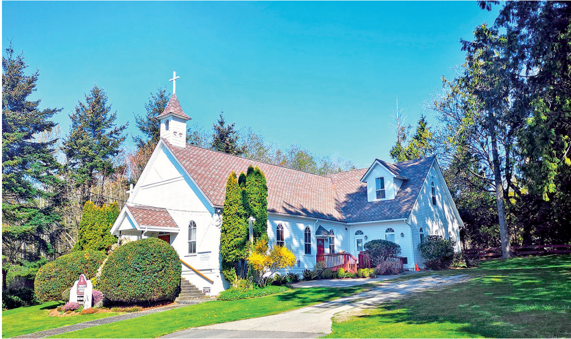
▲ Trinity Community Lutheran Church, one of Point Roberts' oldest buildings, is in danger of collapsing and needs $200,000 in repairs.
