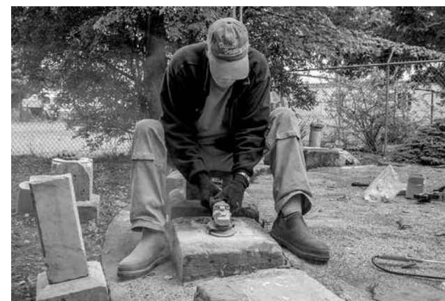
In general, power tools aren't used during cemetery restorations, according to Marion "Mick" Hersey, National Historical Preservationist. However, exceptions are sometimes made. Here, Roy Harlson grinds away old mortar from a base stone which had been combined with an unmatched headstone in a memorial corner created in the corner of Sequim Pioneer Memorial Park.
