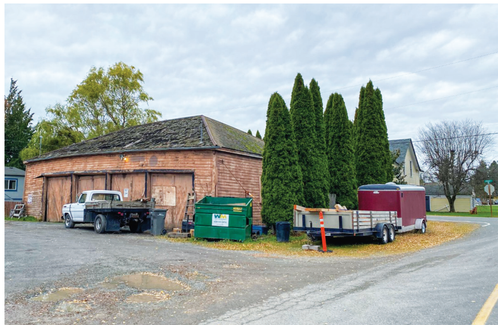
WILL THIS CHANGE BE CONTROVERSIAL? – Kate and Brandon Atkinson have an application in to the Town of La Conner to build a 20-unit apartment building on the corner of Center and Fourth streets. A conditional use permit must be approved for the proposed 14 long term units and six short term dwelling spaces.
